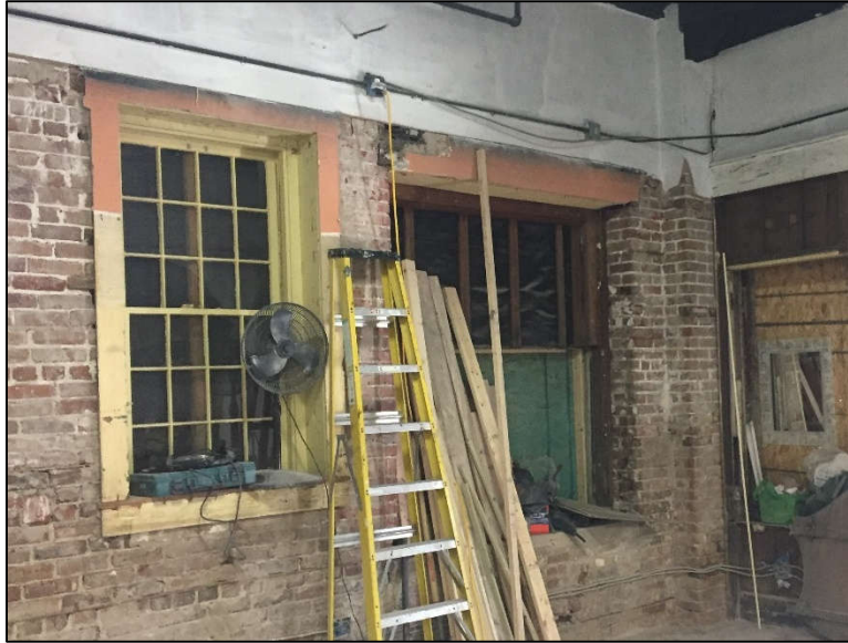
Figure 8: Interior of southeastern corner of subject property storefront, showing historic openings revealed by interior demolition.
