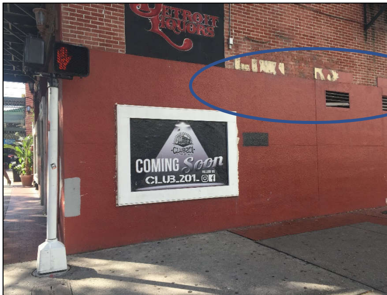
Figure 7: Existing east elevation. Note lintels of enclosed windows above stucco, circled in blue.
